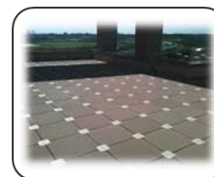
Loose-Laid Paver System
